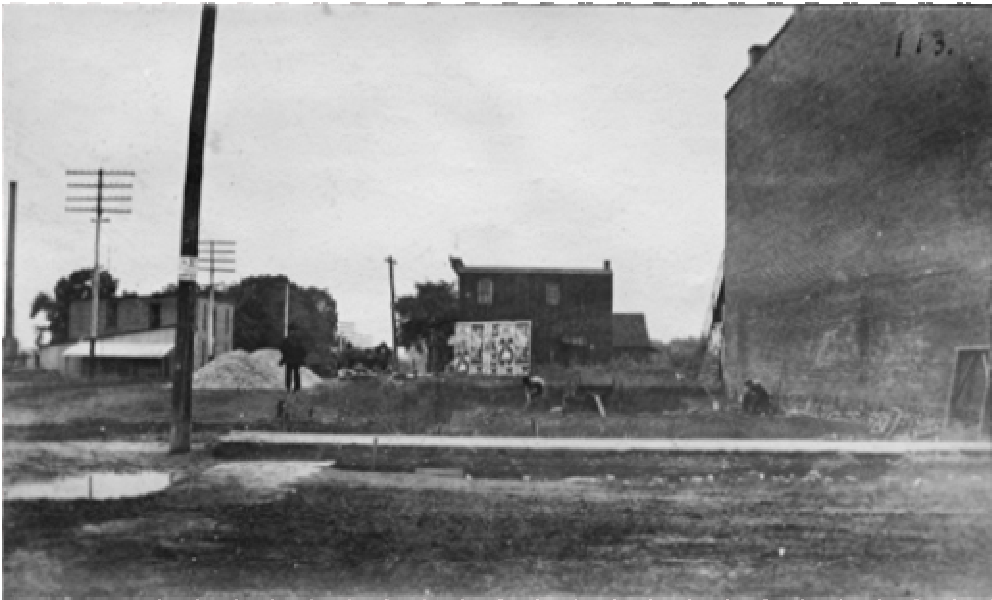
Northeast corner of Main and Palmyra streets cleared for construction of new Peoples Bank circa 1911
