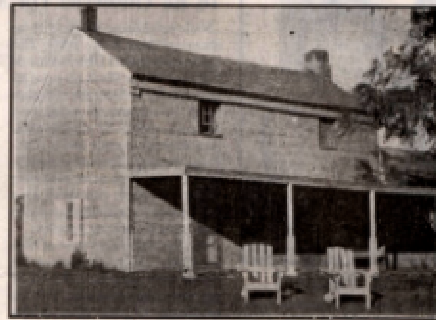
The old inn at Cincinnati Landing after restoration.
